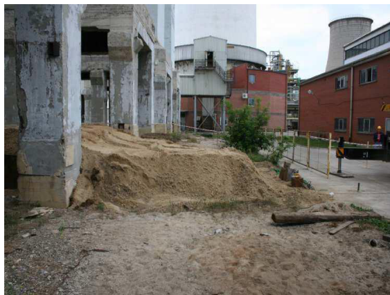
Fig. 16. The damping layer formed as a pile of sand.
