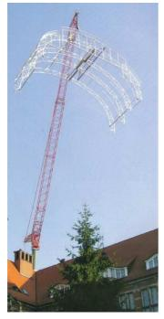
Fig. 19. Transferring glazed roof framework from the assembly site onto the Hevelius Courtyard (Cywiński, 2012).
